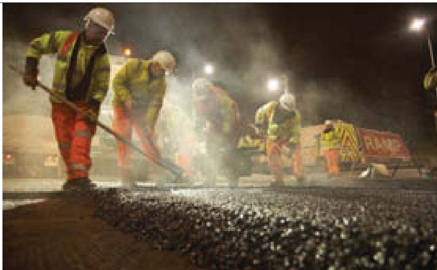
Ongoing work to repair our roads.
