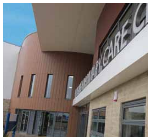
HOUGHTON-LE-SPRING URGENT & PRIMARY CARE CENTRE, SCAPE FRAMEWORK
