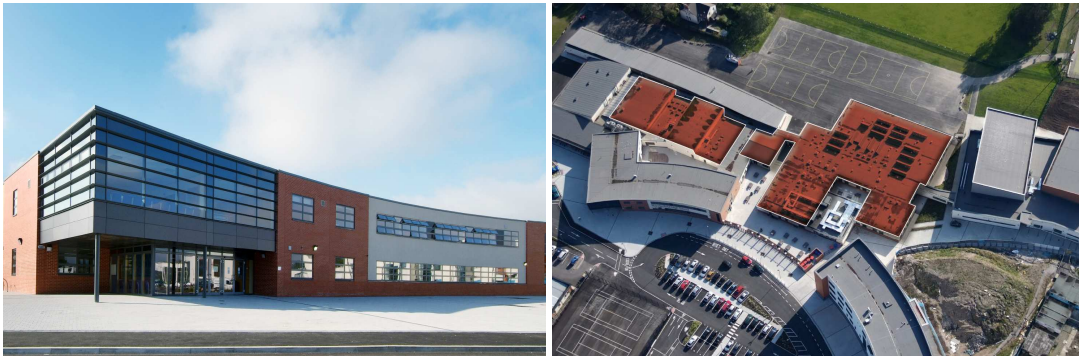
Macclesfield High School – a third is refurbished (in red), while the rest is new build, although you cannot tell which is which
